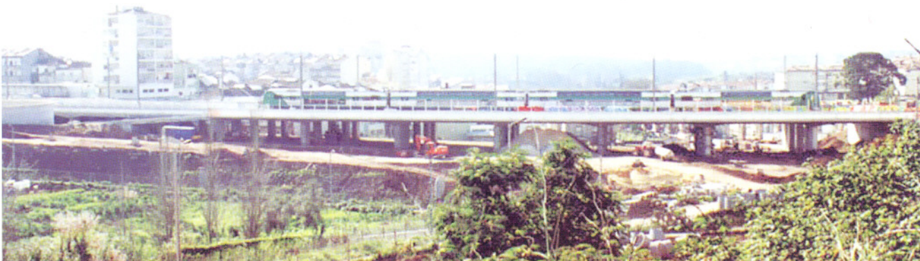
Vista geral do lado Norte General view of the North side
